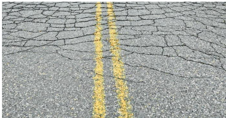
Figure 6 Cracking (Source- www.sidenote.news )
