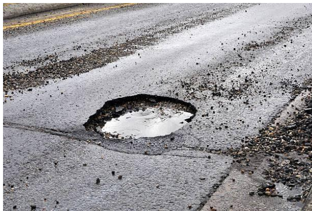
Figure 3 Pothole (Source- www.meonok.com )
