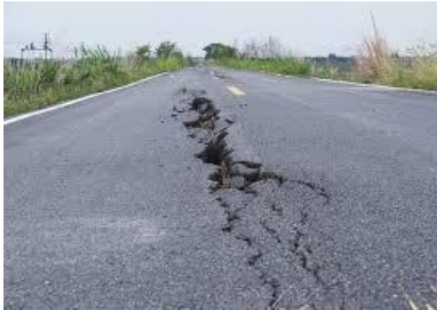
Figure 7 Upheaval (Source- www.superiorasphaltlc.com )
